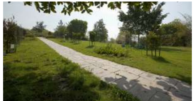
Fig.5. Use of fly ash bricks and concrete in making pathways.
