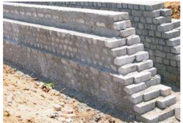
Fig.4. Bricks made using fly ash.
