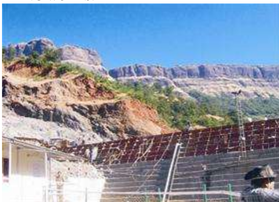
Fig.6. Road Embankment made using fly ash.
