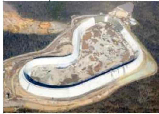
Fig.8. Ameren's Taum Sauk hydroelectric plant.
