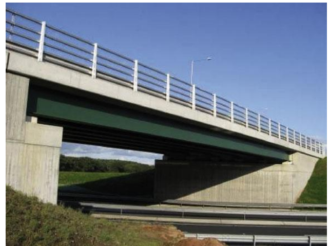
Fig 2: Plate Girder Bridge
